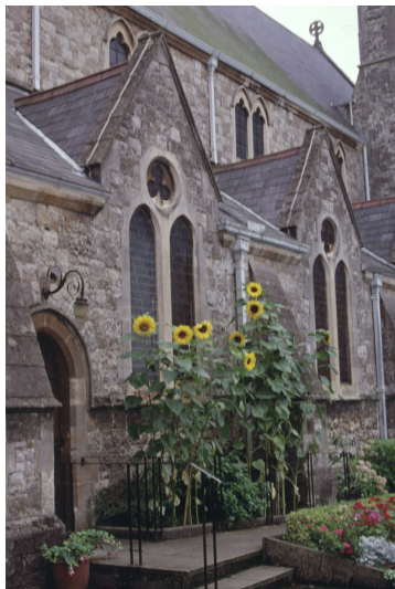
Exterior of the nave and north aisle
